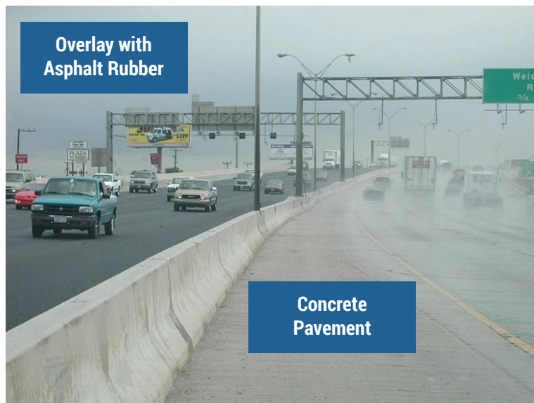
Figure 3. Overlaying existing concrete pavement in San Antonio, Texas with RMA (porous friction course) resulted in better skid resistance, and less spray in wet conditions after (G. B. Way et al., 2011)
